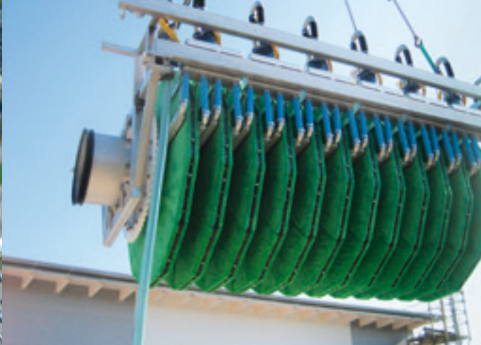
Lahr wastewater treatment plant, installation of a new pile cloth filter
