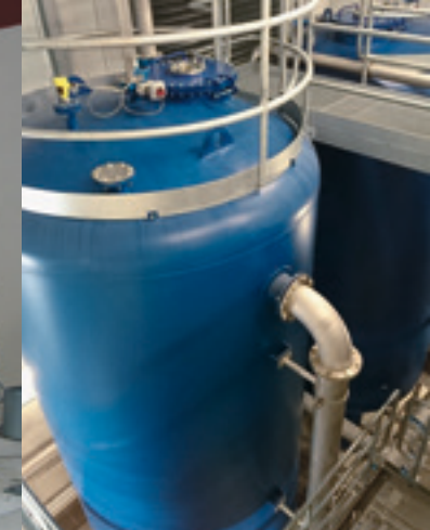
Westerheim wastewater treatment plant, GAC filter
