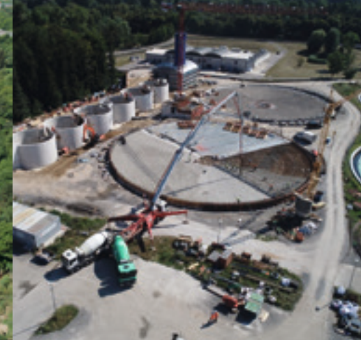
Karlsruhe wastewater treatment plant, advanced treatment stage under construction
