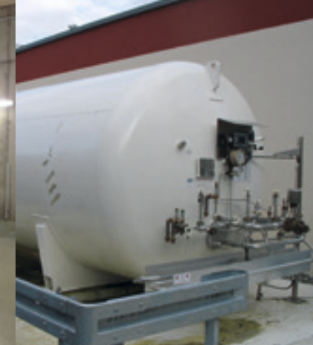
Eriskirch wastewater treatment plant, oxygen tank for the ozone system
