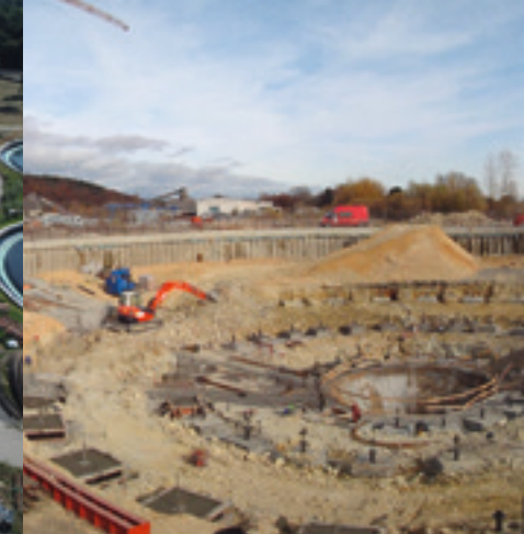
Steinhäule wastewater treatment plant, new sedimentation tank of the advanced treatment stage under construction
