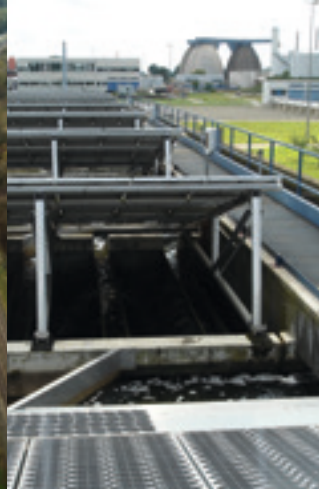
Mannheim wastewater treatment plant, filter with GAC
