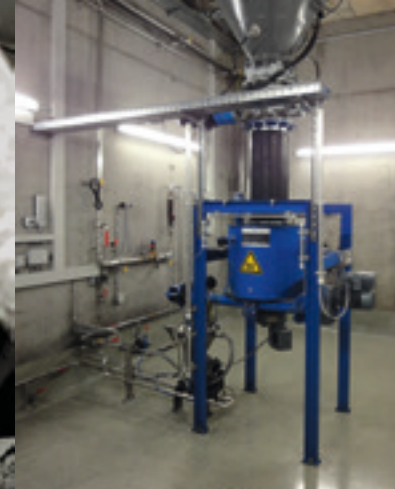
Kressbronn wastewater treatment plant, PAC dosing system
